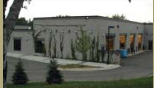
Looking for a way to generate additional income, DARTS started its own business. Dakota Area Resources and Transportation for Seniors built this vehicle maintenance facility that currently services 400 vehicles annually for other nonprofit organizations. DARTS recently earned national recognition for its business model from the Yale School of Management and the Goldman Sachs Foundation.
